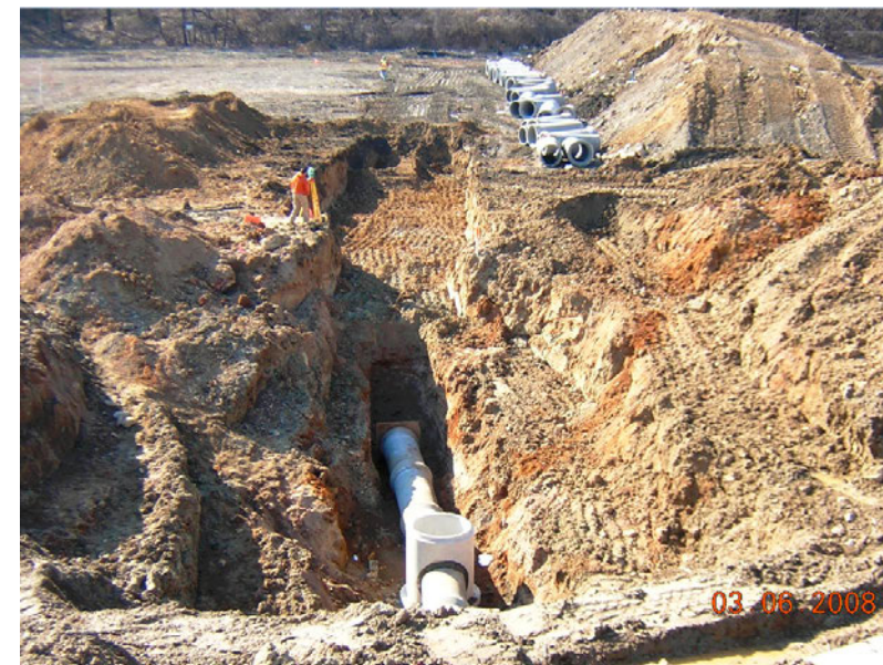
Sewer trench construction Image courtesy of Tetra Tech – 16 March 2008
